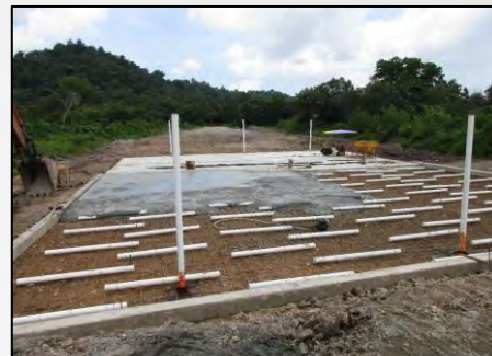
Concreting RC slab
