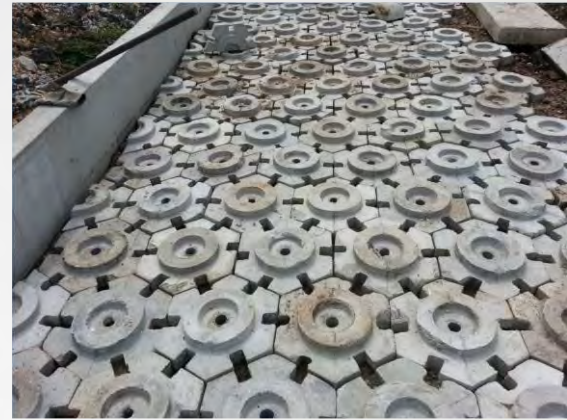
Fig 3.4 Pilot road project using StormPav green pavement at Kg Mang, Samarahan, Sarawak, funded by JKR Sarawak [in progress]
