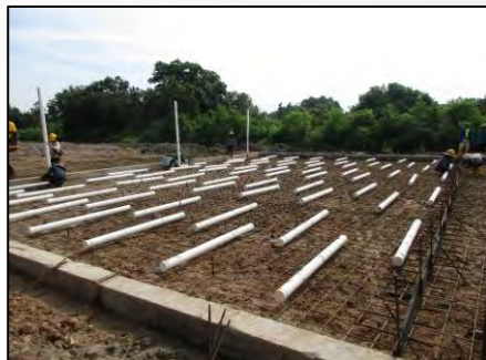
Reinforcement, Formworks and Laying of UPVC pipe
