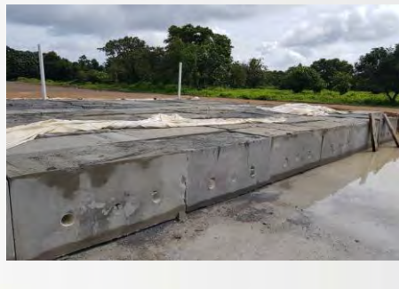
Arrangement of lightweight foam concrete on site
