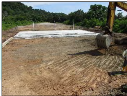
Surface Preparation for RC Slab
