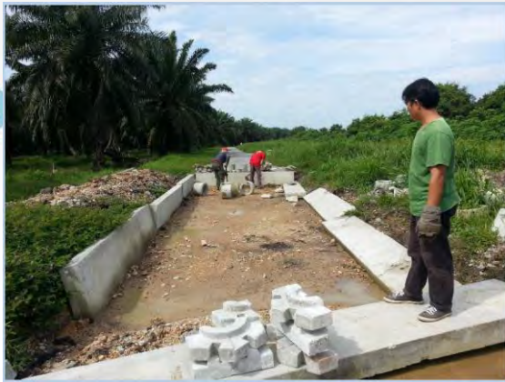
Fig 3.4 Pilot road project using StormPav green pavement at Kg Mang, Samarahan, Sarawak, funded by JKR Sarawak [in progress]
