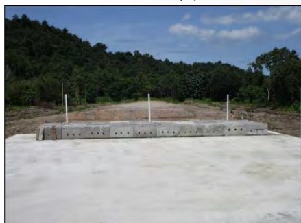
Foam Concrete Blocks installed
